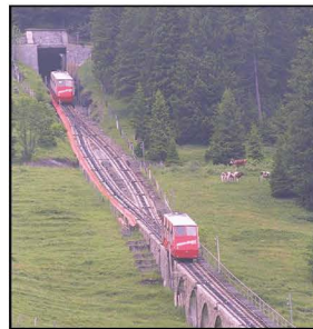
(c) Passenger incline (Müren, Switzerland)
