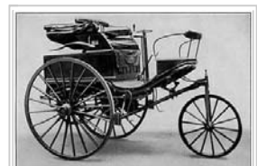
The Benz Patent-Motorwagen Number 3 of 1888, used by Bertha Benz for the first long distance journey by automobile (more than 106 km or sixty miles)
