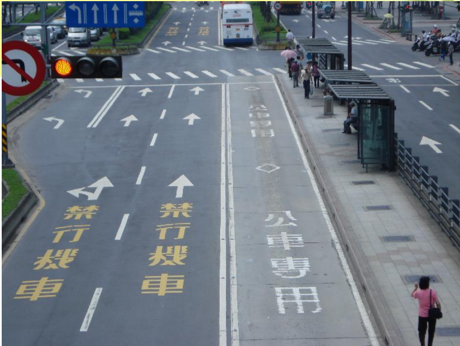
Bus Lane Markings for BRT System in Taipei. Department of Transportation Technology and Management
